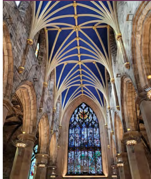
Plaster vault in nave
